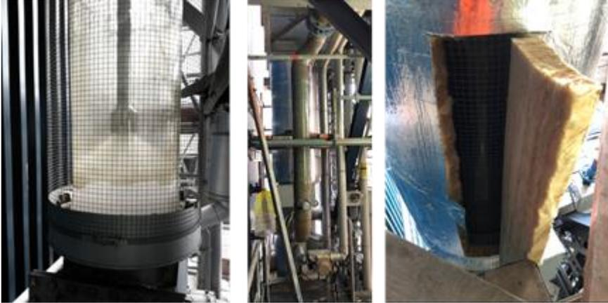
**Figure 2. Turbulent spray scrubber used for the tests of NO<sub>2</sub> removal. left: before insulation, middle: after complete insulation right: observation window in the insulation**
